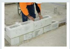
Maximum span between control joints is 8m
