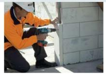
Use type 17 wood screws for fixings
