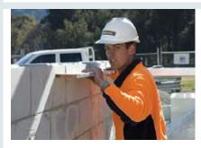
Check blockwork for plumb and straight each course
